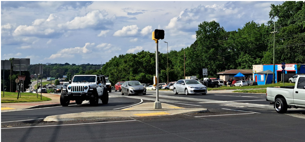
Figure 9-2: Right Turn Slip Lane on South Cobb Drive at Austell Road
